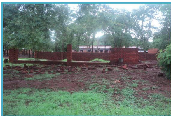
Picture 5.9: Ongoing construction of residential houses for the Liganga primary school teachers.
