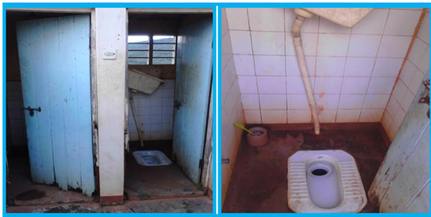
Picture 6.8: The Epsom Company's washrooms for the workers.
